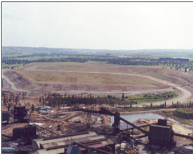
Figure 4.8: Collection and discharge channel at closed Apirsa tailings pond
