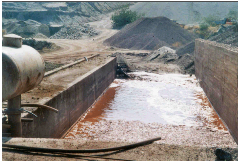
Figure 3.49: Dewatering of tailings in concrete basins [110, IGME, 2002]
