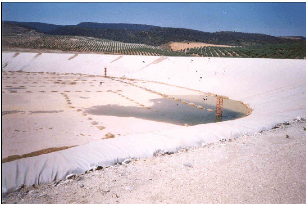
Figure 3.59: New strontium TMF with a synthetic liner and decant towers [110, IGME, 2002]
