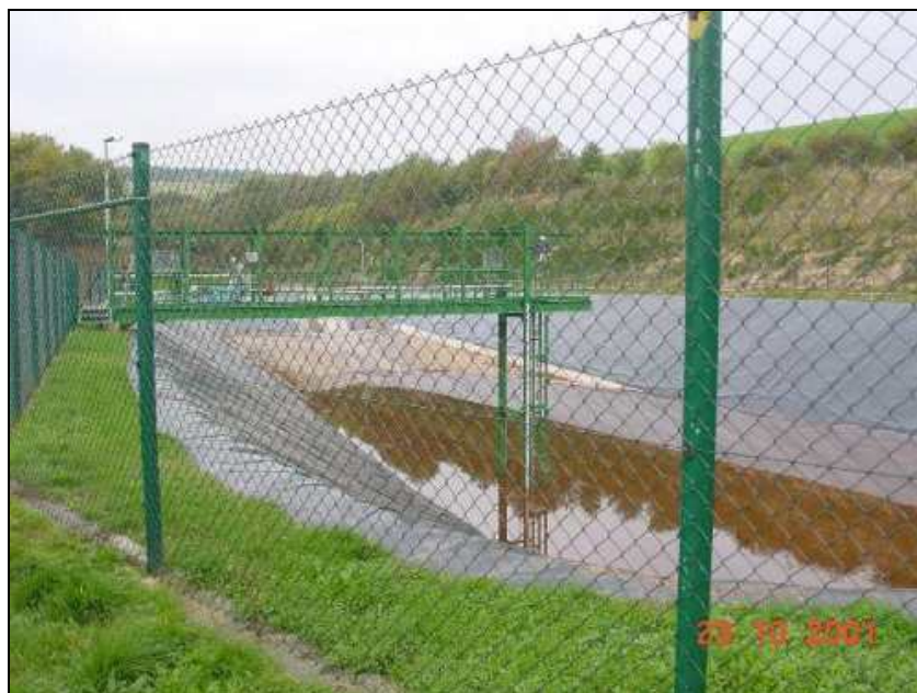
Figure 3.75: Water retention basin of German potash mine
