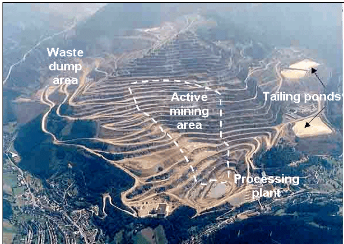
Figure 3.33: Steirischer Erzberg [55, Iron group, 2002]
