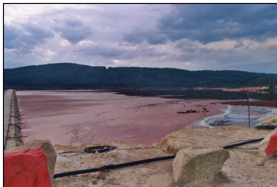
Figure 2.32: Example of a beach at an alumina refinery’s red mud pond
