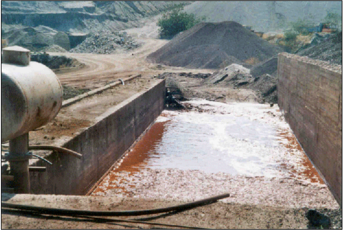
Figure 1.24: Example of a small tailings settling basin
