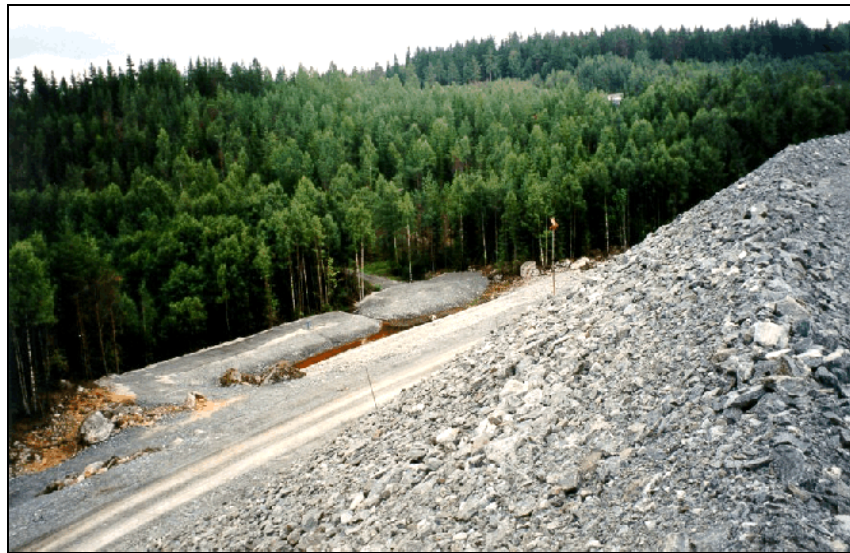
Figure 3.22: Ditch for collection and flow measuring of seepage water alongside the dam [66, Base metals group, 2002]
