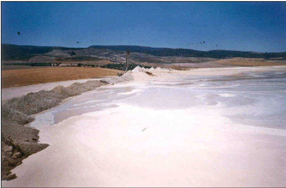
Figure 3.58: Old strontium TMF with tailings in structural zone [110, IGME, 2002]
