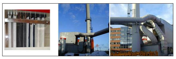
Figure 4.10: Bag filter units; inside (l.) and outside (m., r.) views [237, HUT, 2003]
