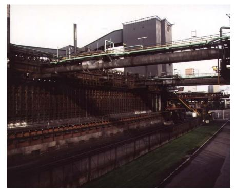
Figure 6.1 : Photograph of a coke oven battery showing the chambers, the coal tower and the coke oven gas collecting main
